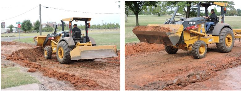
**Figure C.11. Excavation and preparation for concrete pavement**
