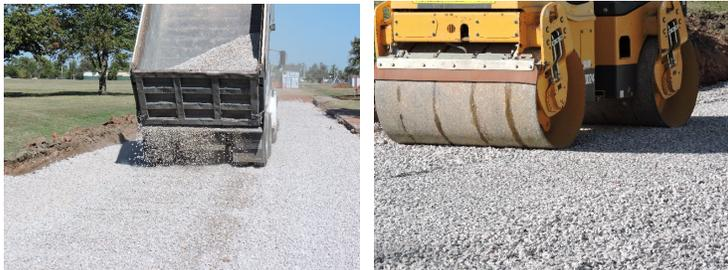
**Figure C.12. Installation and compaction of aggregate base for concrete pavement**
