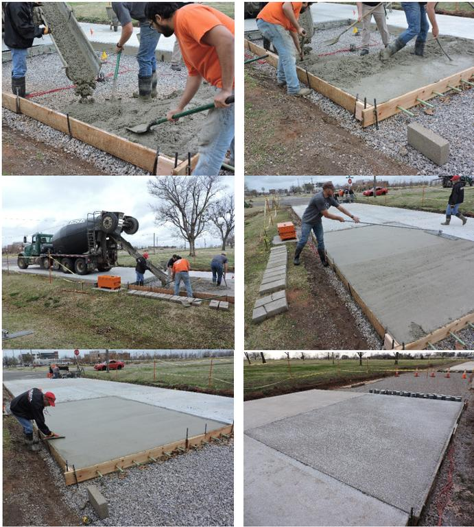
**Figure C.15. Concrete placement and consolidation**
