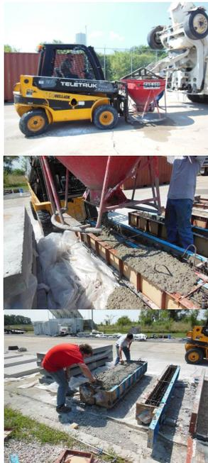
**Figure C.21. Concrete beam construction procedures**
